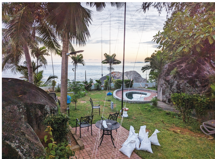
PHOTO 2: Many antennas can be packed into a small space but watch out for inter-station interference, Note the rubble bags filled with sand to act as guying points.
