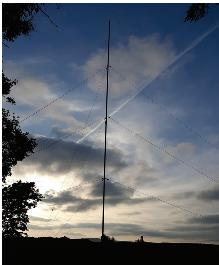
PHOTO 2: Nick, G4FAL's LF vertical antenna.
